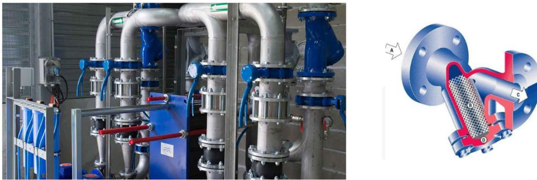
Gambar 1. 1 Strainer Valve Type Y
