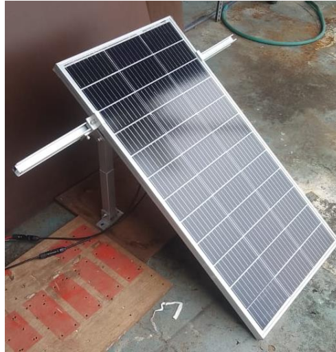
Gambar III.12 Mounting Panel Surya
